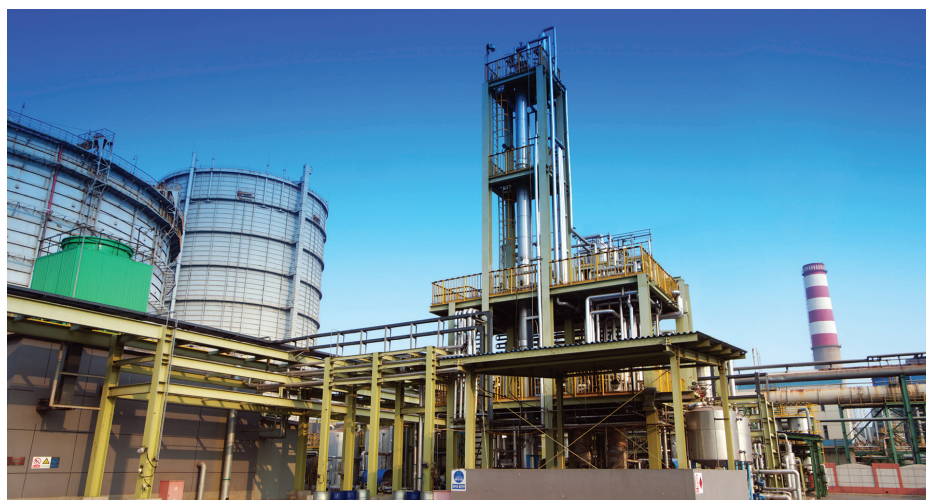
At waste-gas-to-fuel plants like this one in China, Jewett's collaborators at LanzaTech use clostridia to produce sustainable fuels.
